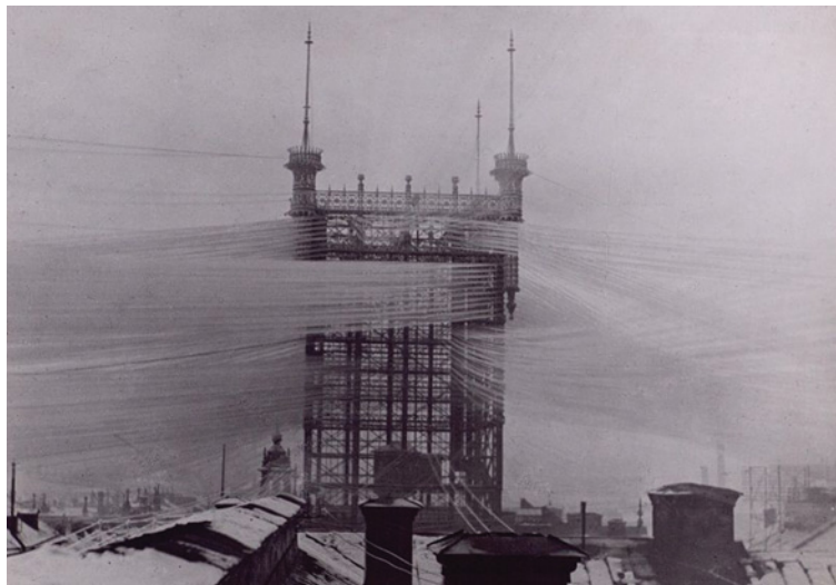
Figure 33.5 A telephone tower in Stockholm, Sweden, with 5000 connected lines. It was used between 1887 and 1913, but the tower stood there until 1953, when it fell down after a fire. www.flickr.com/photos/tekniskamuseet/6838150900/in/set-72157629589461917
